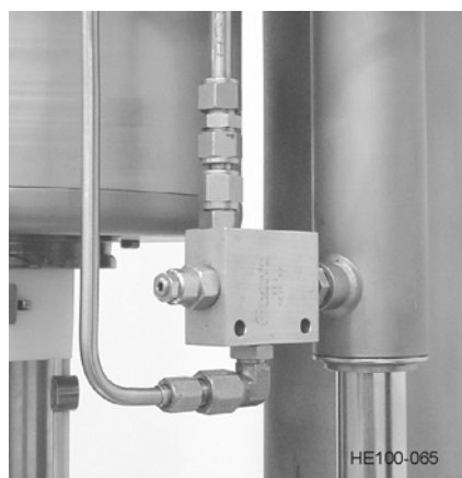
Figure 20 - Balance Valve
